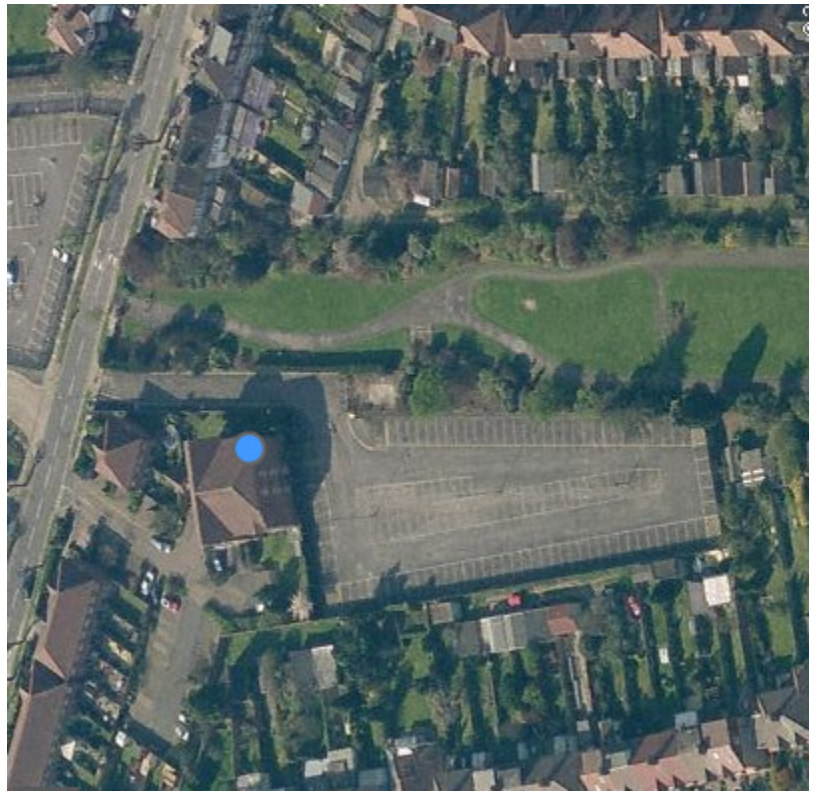
M65 Car Park adjacent to Kendor Gardens: Site Views
